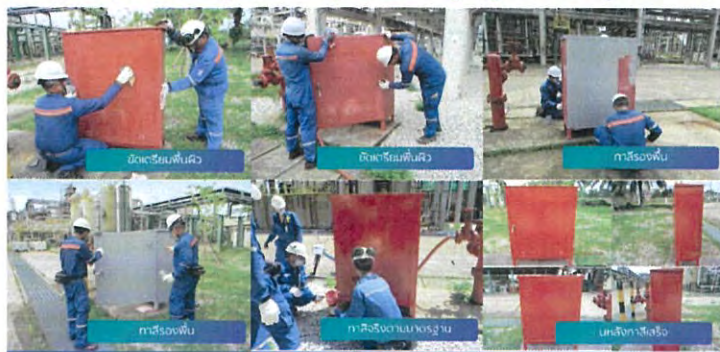
AM/PM activities "Repair and painting fire hose box"
